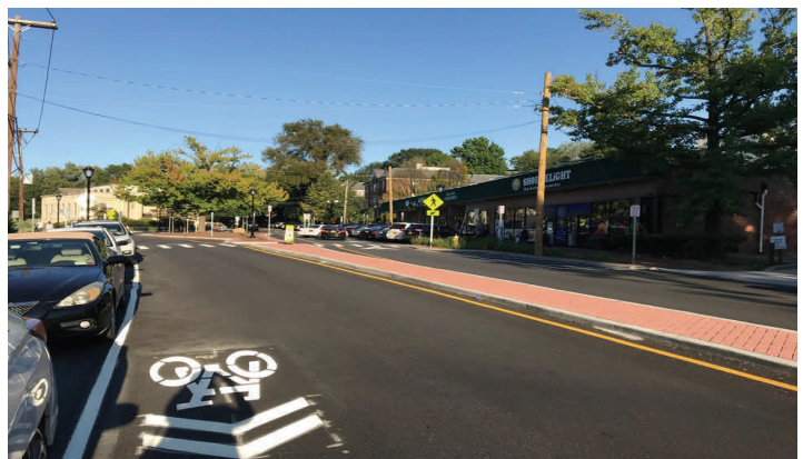
“After” looking at the USPS Post Office, 1 Welwyn Road, and the completed project, with a constructed median, highly visible crosswalk and bicycle sharrow.
